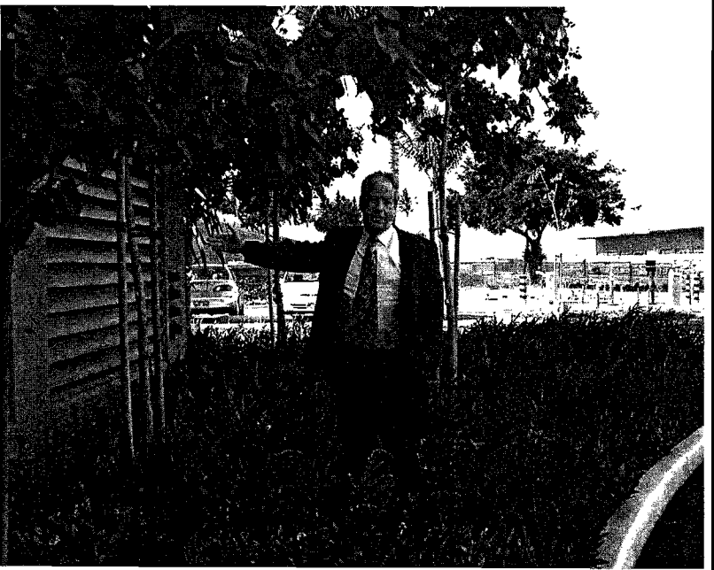
The JABSOM back-up generator is in the building closest to the ocean. The fencing on the right is a drainage canal to the ocean, 300 yds away.
